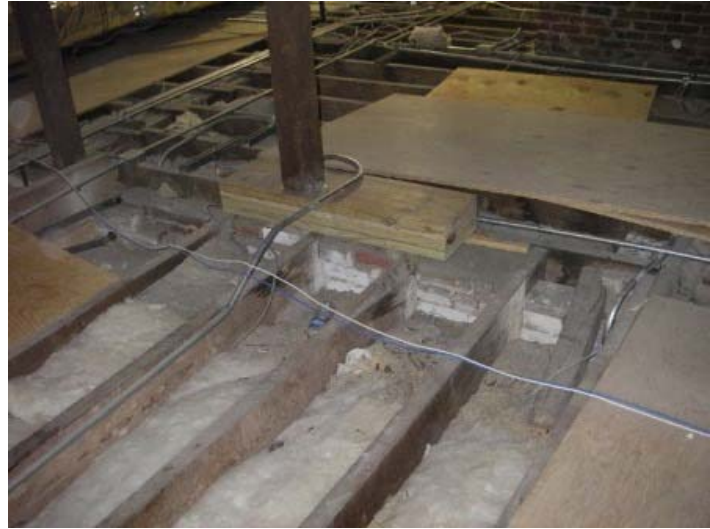
Figure 31: Existing Wood Joist Layout
